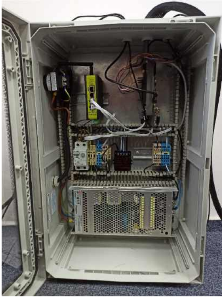
Figure 13: Control cabinet of the exoskeleton.
